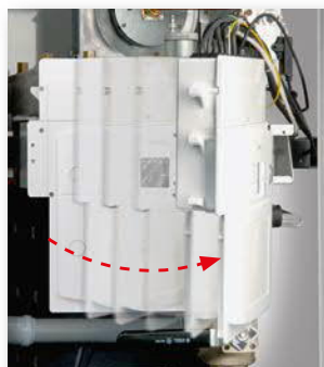
The control panel can be opened to facilitate maintenance
